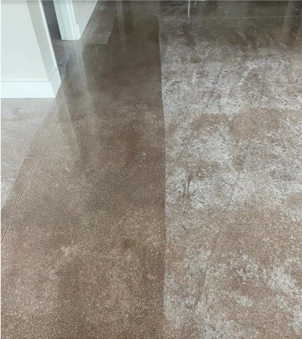
As the moisture/water evaporates, it can leave mineral salts on the surface of the concrete, which resembles grainy dirt with a white-ish appearance. Efflorescence has more to do with the concrete mix ingredients, placement, how much water was used during pouring, and the temperatures and humidity leading up to the finish work than it does with the concrete sealing/polishing process.
